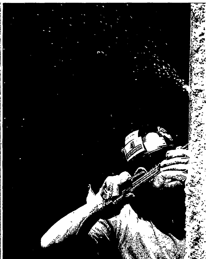
In August, John Linehan of Rochester Rigging & Erectors welds tube steel during construction of the narthex, or gathering space.
