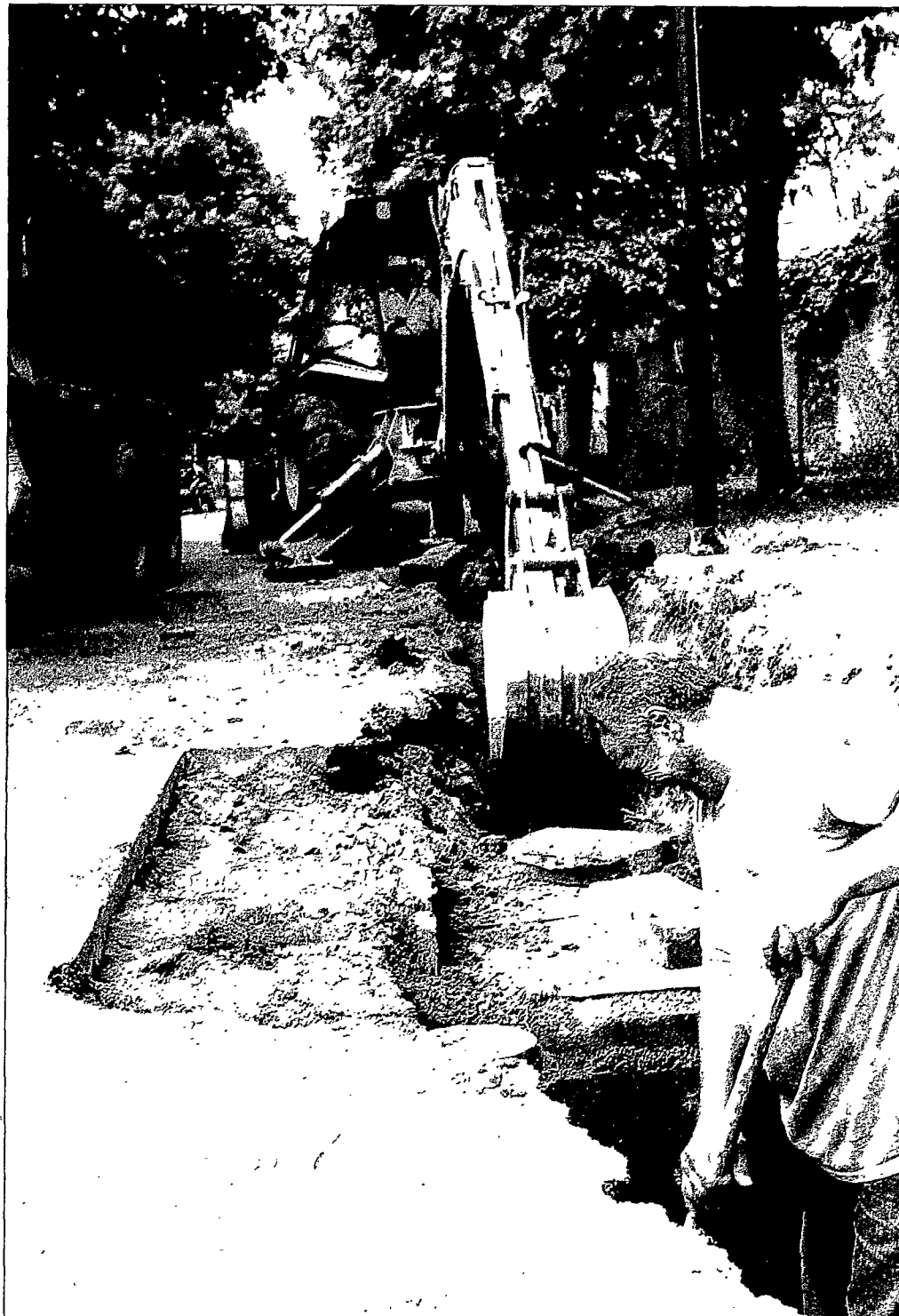
Alex Ingavo, foreman for Falcone Concrete, works with Bergman Associates to replace curbs on Pembroke Street in Rochester. Bergmann is covered by Rochester's living wage law, which mandates a minimum wage for contractors with the city government.
