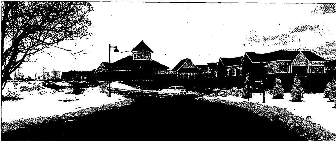
The new Sisters of St. Joseph Motherhouse on French Road in Pittsford.
