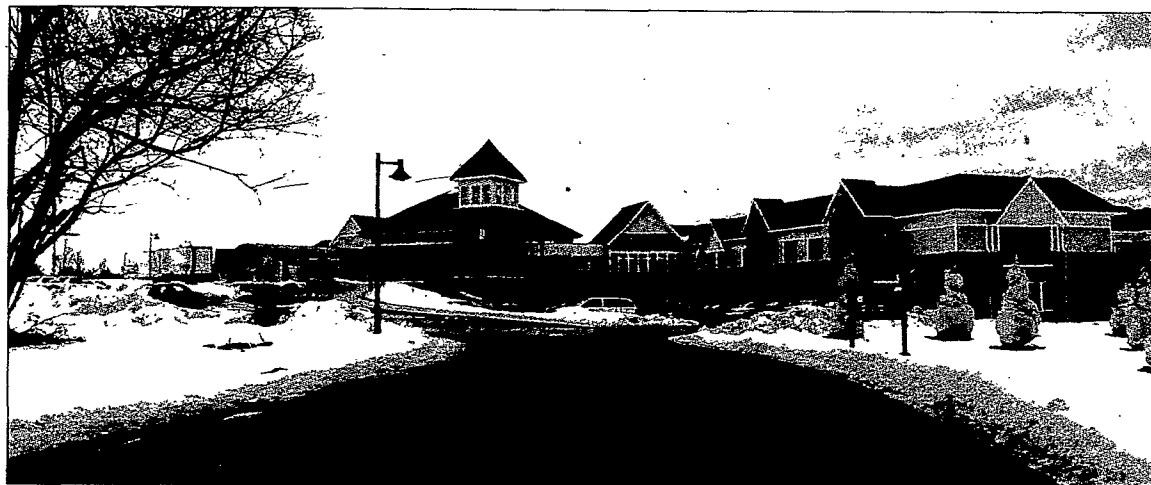
The new Sisters of St. Joseph Motherhouse on French Road in Pittsford.
