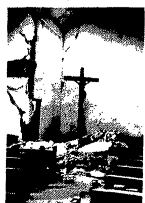
Chapel at Ende, Indonesia, after the earthquake
