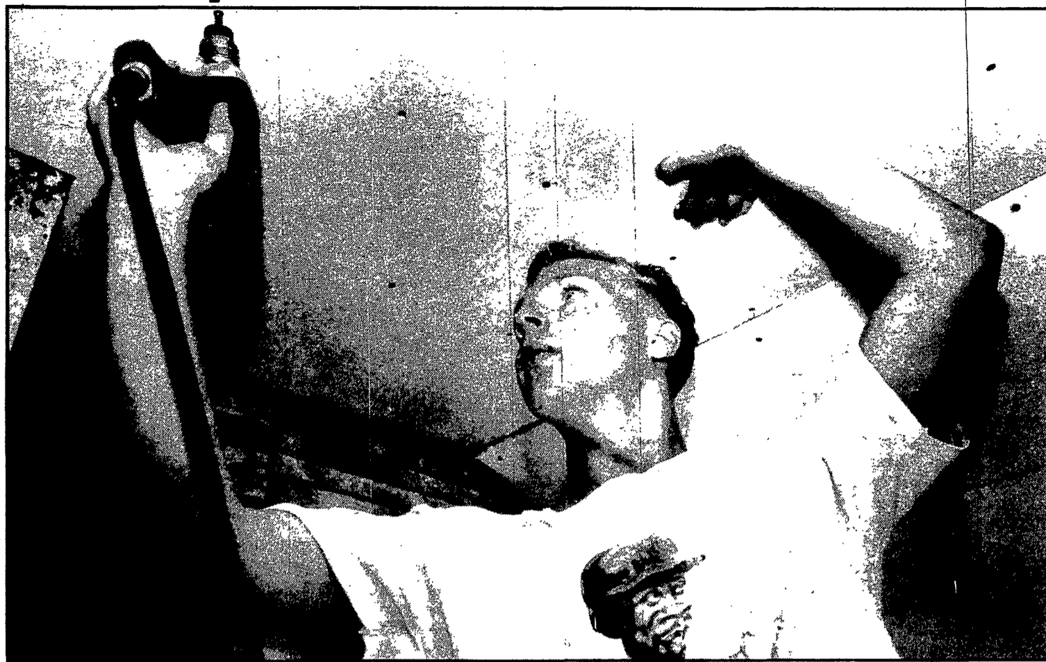
Group Work Camp volunteer Ryan Adelman from Lancaster, Pa., concentrates on fastening drywall to an upstairs room in a Seneca Falls home.
