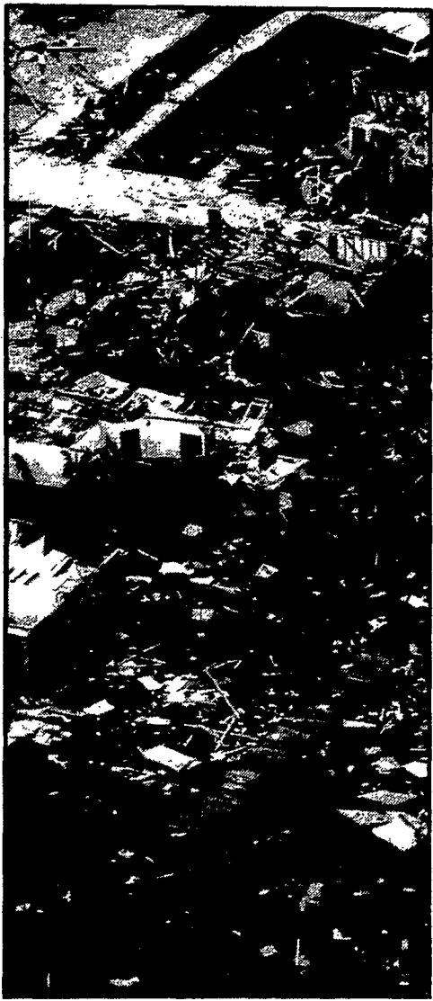
AP/Wide World Photos This aerial view shows the damage caused to a subdivision in LaPlace, La. after Hurricane Andrew produced a tornado on Aug. 26.
