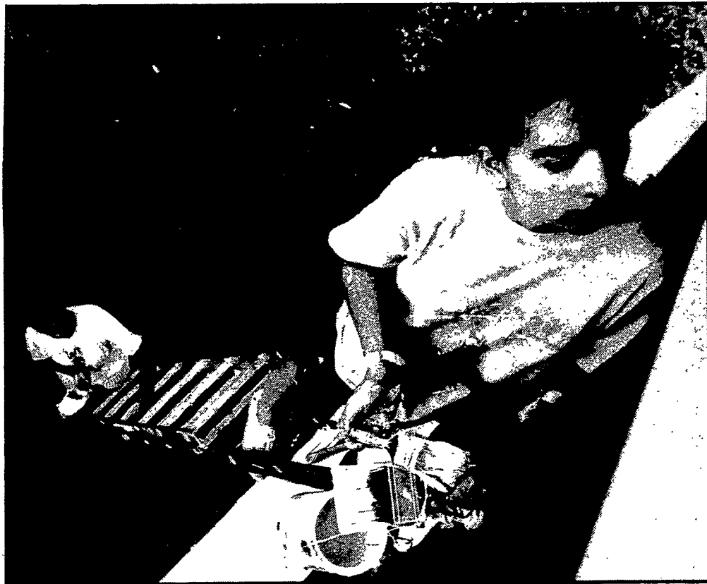
High atop a ladder, Michelle Fairbrother takes a second to assess her work on the awning around the roof.
