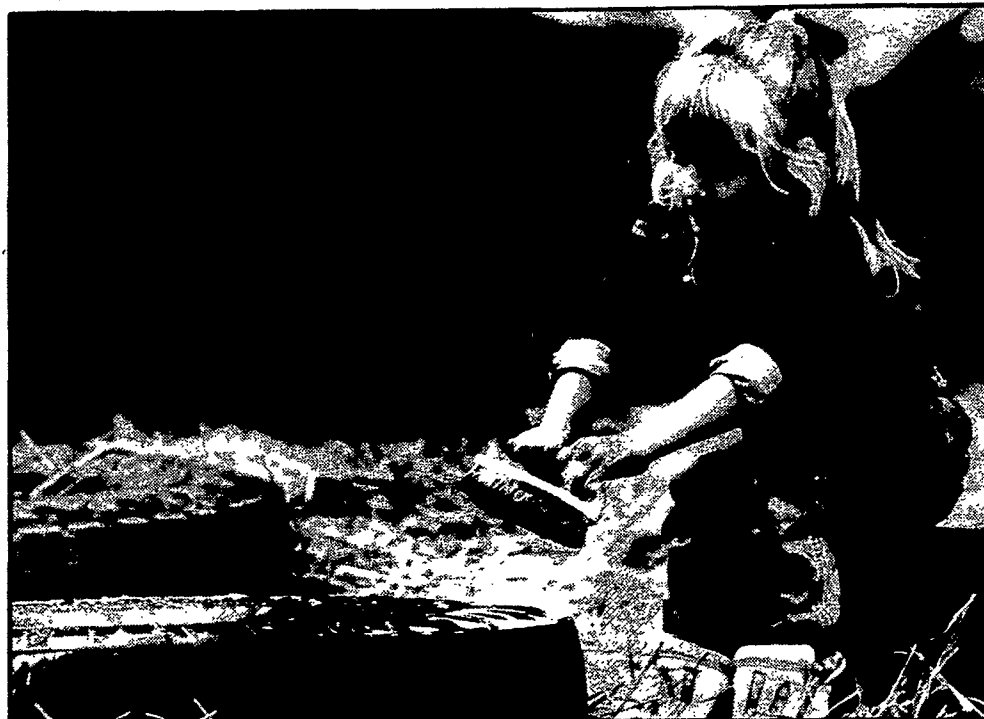
TIRING JOB — Six-year-old Megan Myers of Hilton was one of some 1,400 volunteers who pitched in to help construct the Parma-Hilton playground last week. Megan got the job of scrubbing down old tires to be used in various parts of the playground.
