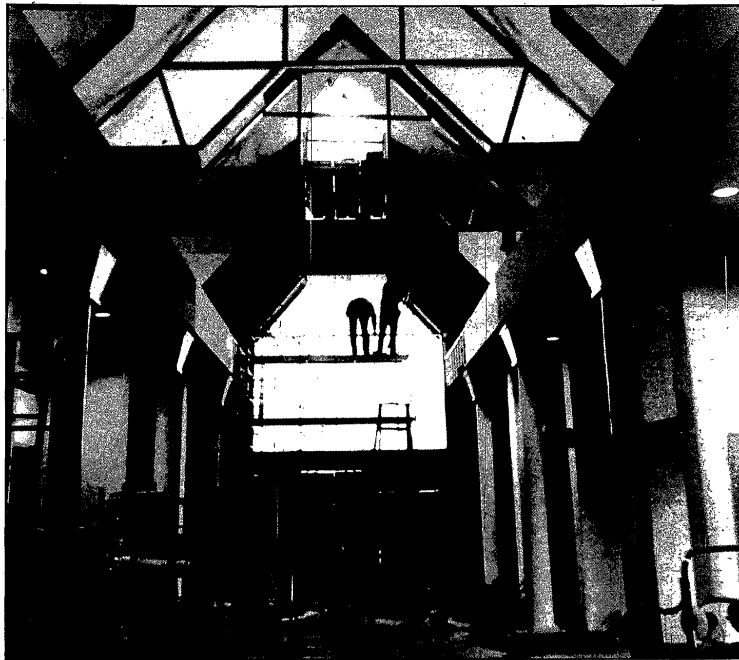
Workers at the International Museum of Photography at George Eastman House finish up construction of the Potter Peristyle. The museum opens to the public Jan. 28 for a celebration of the 150th anniversary of the birth of photography.
