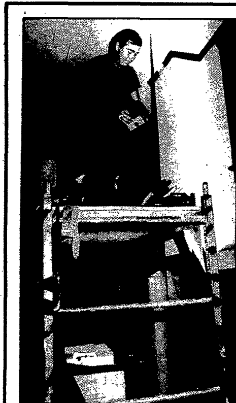
Larry Mitchell of Rochester's Blackman and Farrell Electric Company installs a new fire alarm system at Nazareth Academy on Lake Avenue.
