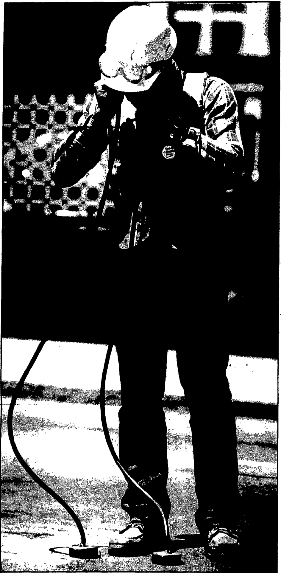
PULSE OF THE CITY — Rochester Water Authority worker Stan Tucker used a large stethoscope last week to listen for a water leak on Platt Street. For an indefinite period of time, said Tucker, 100,000 gallons of water a day went down the city's drains.
