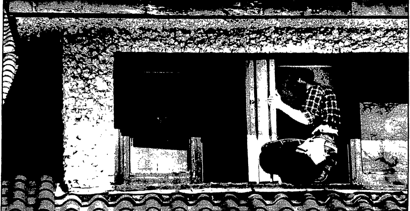
Peter Reis, supervisor, finishes a wall that divides two newly created rooms.
