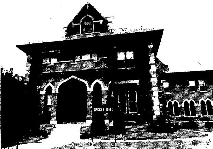
The new Becket Hall on Gregory Street.
