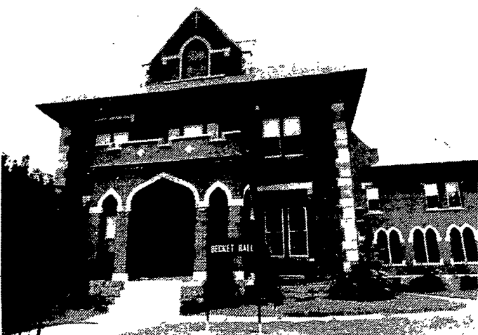
The new Becket Hall on Gregory Street.
