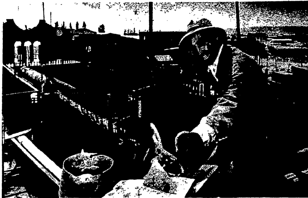
After nearly 17 years, Justo Gallego, 57, says it will take him another four years to complete the church he plans to turn over to the town of Mejerada del Campo near Madrid, Spain. The former seminarian is the architect, financier, and sole construction worker on the project.
