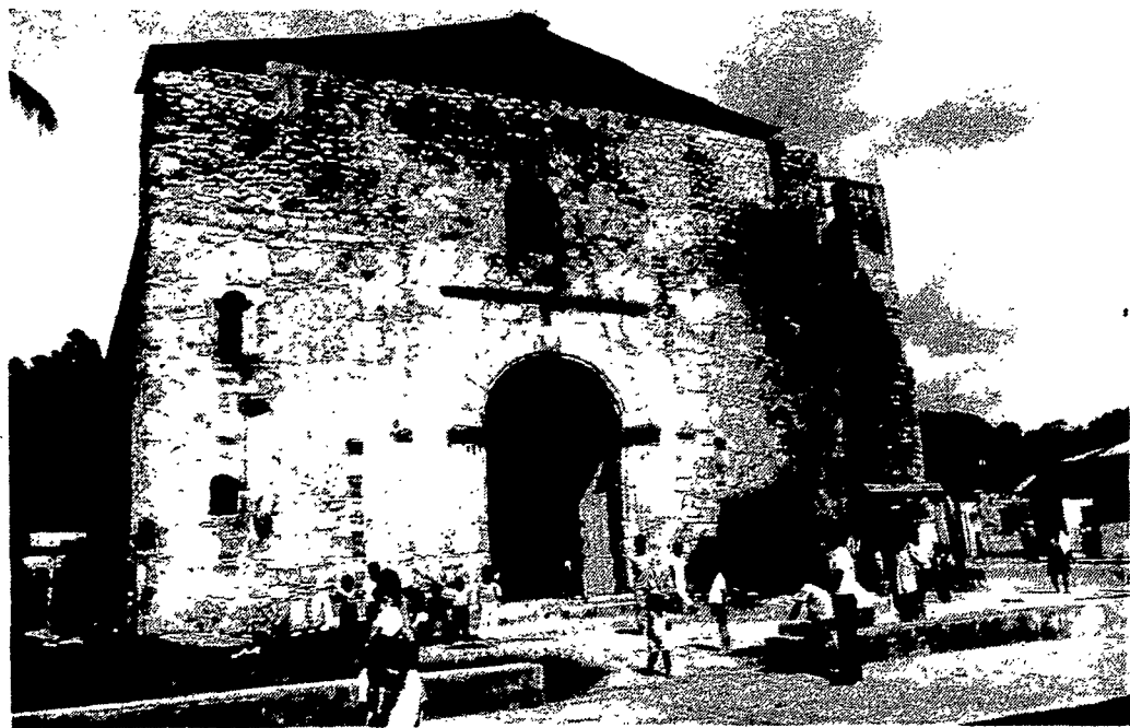
St. Dominic Church in Oxolotan, built in the 16th century by Dominican missionaries, features stone walls six feet thick.
