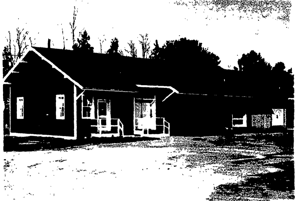
The outside of the church.
