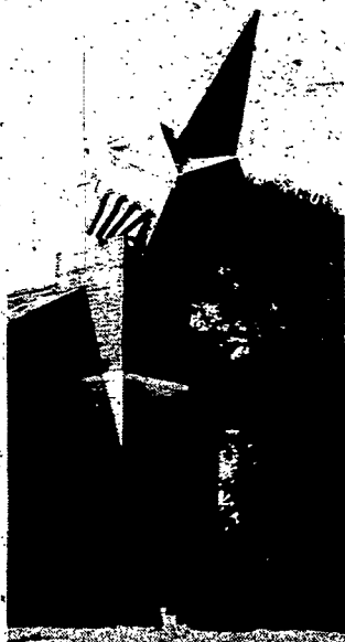
The steeple topples.
