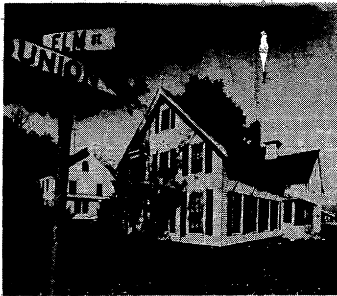
PRE-FINISHED ALUMINUM SIDING restored this old colonial-style house to its original beauty, and aluminum trim preserved special architectural details around windows and doors. Insulation installed behind the panels helps reduce fuel use. With warranties of up to 40 years, aluminum siding has been repays its original cost by eliminating need for repainting.
