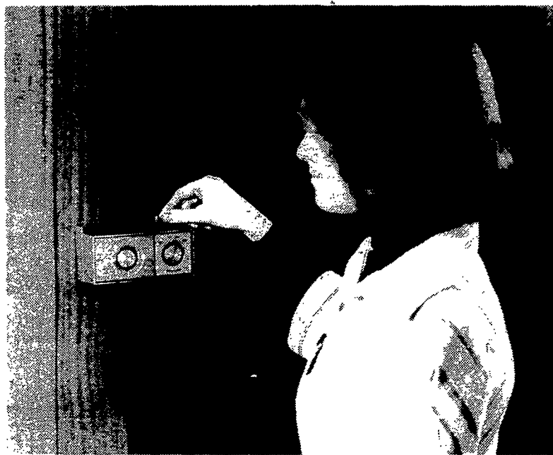
Automatic clock thermostats help conserve energy.
