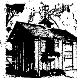
WOODEN UTILITY BLDG
