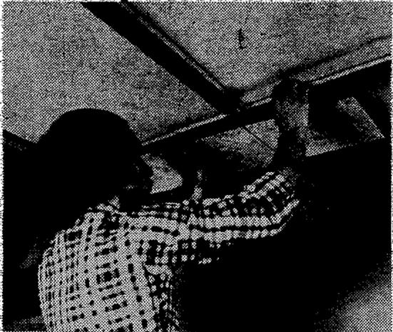
INSTALLING A TILE CEILING is a lot faster and simpler now, thanks to new techniques like Armstrong's Integrid System. Lightweight metal furring channels replace old-fashioned wood strips—and instead of stapling the tile, you simply lock it into place with a cross tee that snaps on to the channel. No special tools are required.
