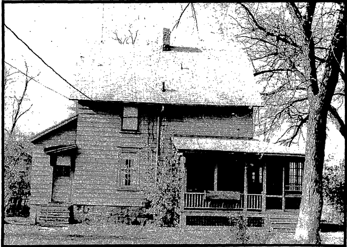
Repairs to this house enabled a mother and her daughter to move into a home of their own.
