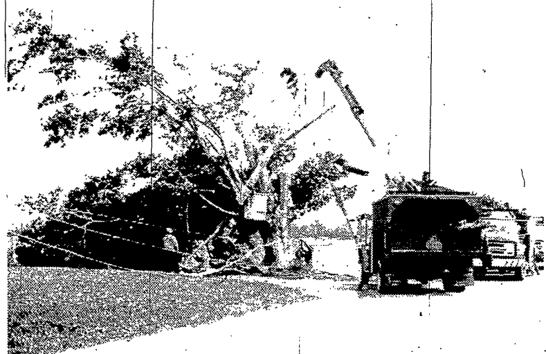
RG&E crews at work restoring electric service.
