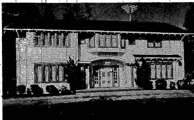
LOOKS LIKE WOOD, but the clapboard look on the exterior of this home is actually vinyl siding with "wood-grained" finish, manufactured by Certain-teed Products Corporation. Vinyl siding is maintenance free, and is guaranteed for 20 years.
