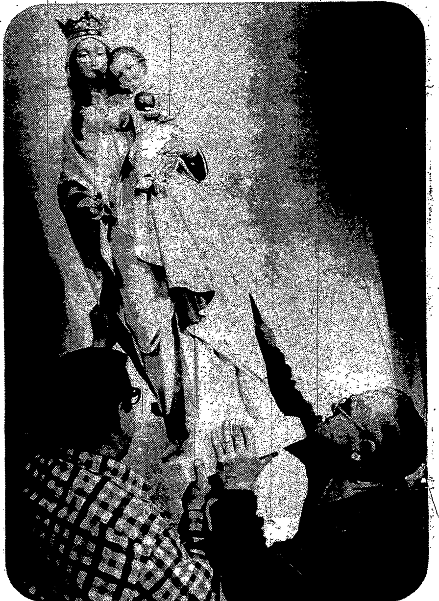
Robert Gates, a member of the parish building committee, and Laurence Koski, supervisor for Welliver Construction Company, lift a statue of the Virgin and Child to its place in the sanctuary.
