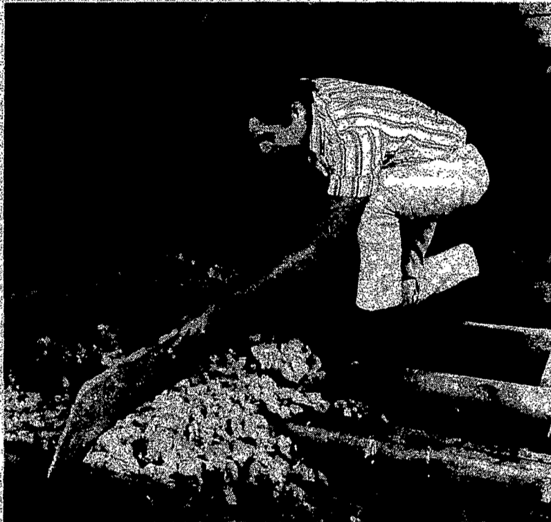
RG&E has prepared a booklet, "If You're Under-insulated, You're Overspending on Fuel." This booklet explains, step-by-step, how to insulate your home. It also includes safety tips and information about different types of insulation.
