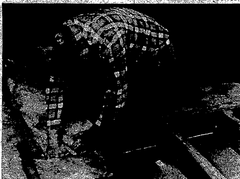
When installing blanket insulation, press the rolls between the crossbeams, starting at one end and unrolling them as you go.
