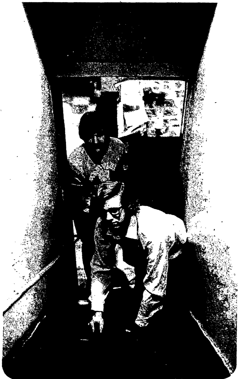
Repairing steps in a low-income home, Greg Smith puts on the tread covers while Michael Jones helps.
