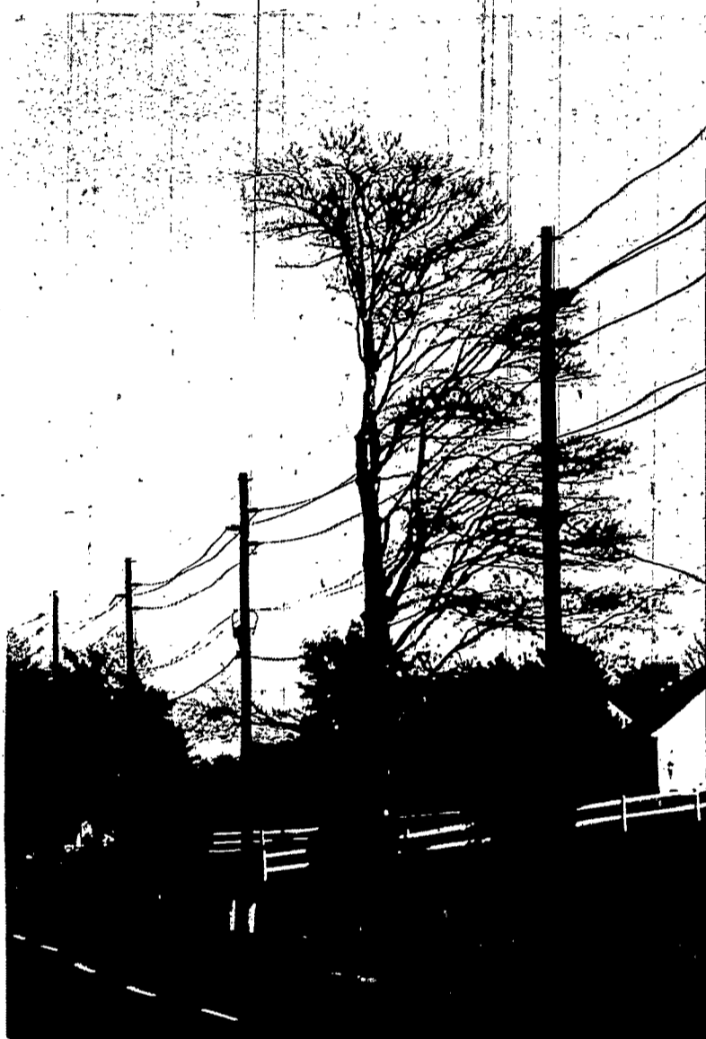
This tree is a hazard to power lines and must be trimmed regularly.
