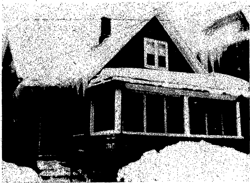
A family of seven moved into this Loomis St. house with the aid of the Bishop Sheen Housing Foundation.
