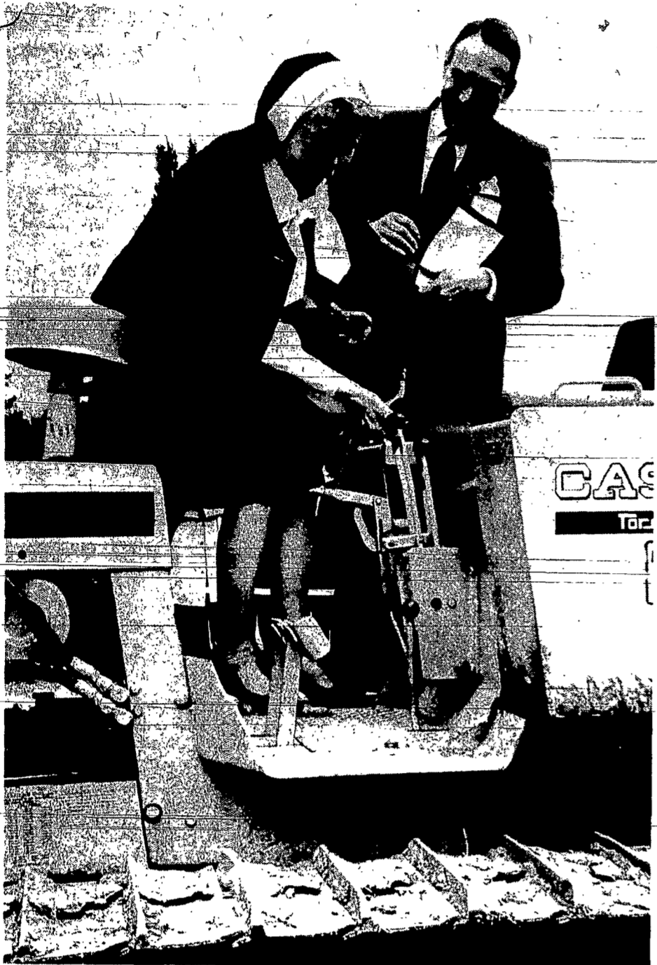
Sister Helen Daniel, SSJ, president of Nazareth College, pushes bulldozer lever at groundbreaking ceremonies for proposed $2.4 million dormitory complex. She is assisted by Peter Barry, Nazareth's board chairman. Dorms will accommodate 320 students.
