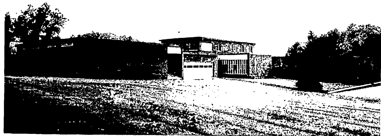
Assumption School of Religion in Fairport is a pioneer institution for CCD instruction. Diocesan CCD planners predict that buildings like this will soon multiply providing day and evening use for parishes which do not have schools or for several parishes at once where the construction was shared cooperatively. As the quality and range of instruction improves larger numbers of public-schoolers are attracted to the programs. Construction of such centers as close as possible to the local public schools aids the efficiency of using released time.
