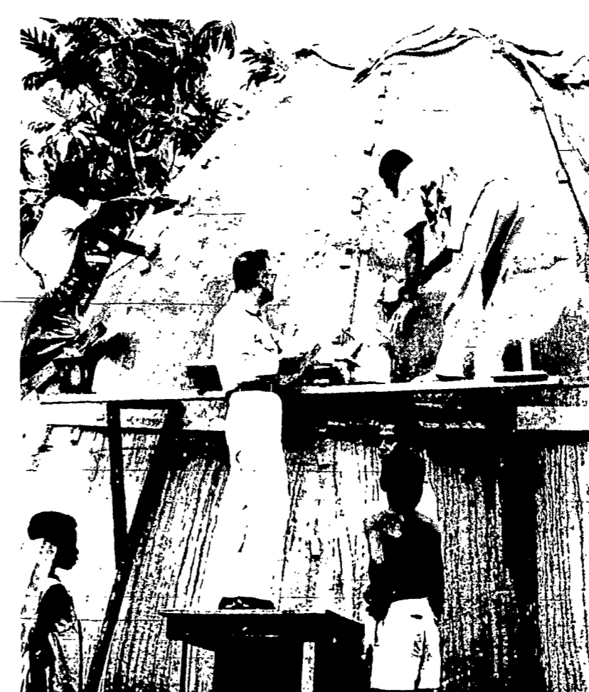
Columban Father Dermot Hurley and his native construction battalion erect low-cost ctesiphon house on Fiji. Whole villages of economy houses have resulted from priest's work.
