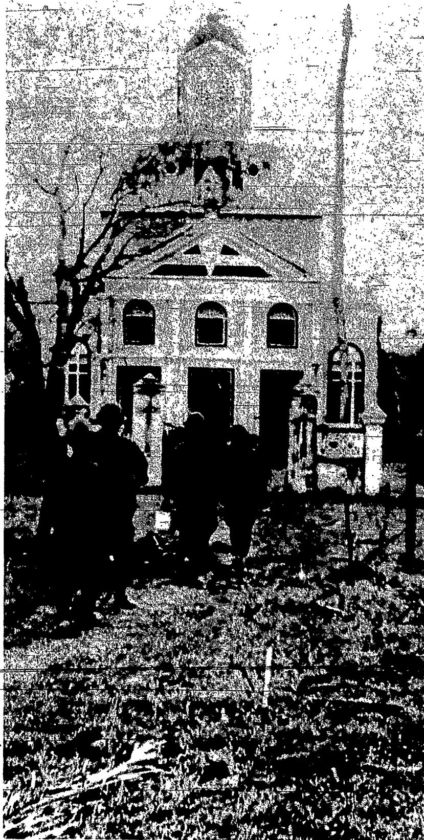
Vietnam — (RNS) — Soldiers of a joint U.S.-South Vietnamese patrol move toward a Roman Catholic church which recently sustained heavy interior damage during an air bombing of Vietcong troops who controlled the forward area.
