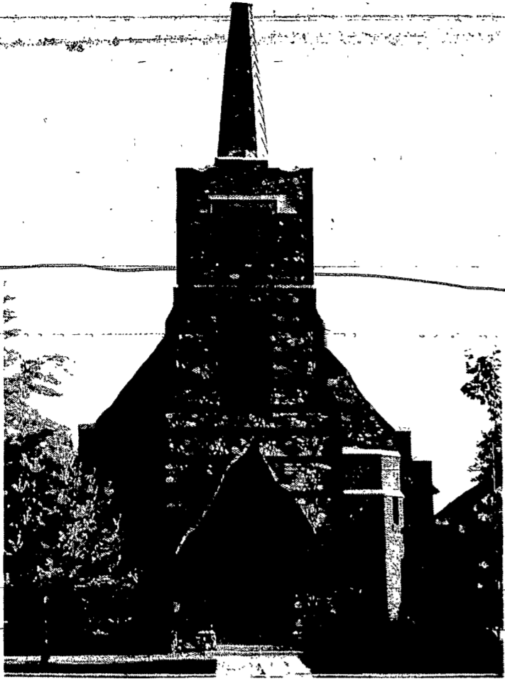
St. John the Evangelist Church, Spencerport, built in 1915 is currently being renovated in interior for centenary of parish. Jubilee Mass will be celebrated Sunday, October 8, at 12:30 noon.
