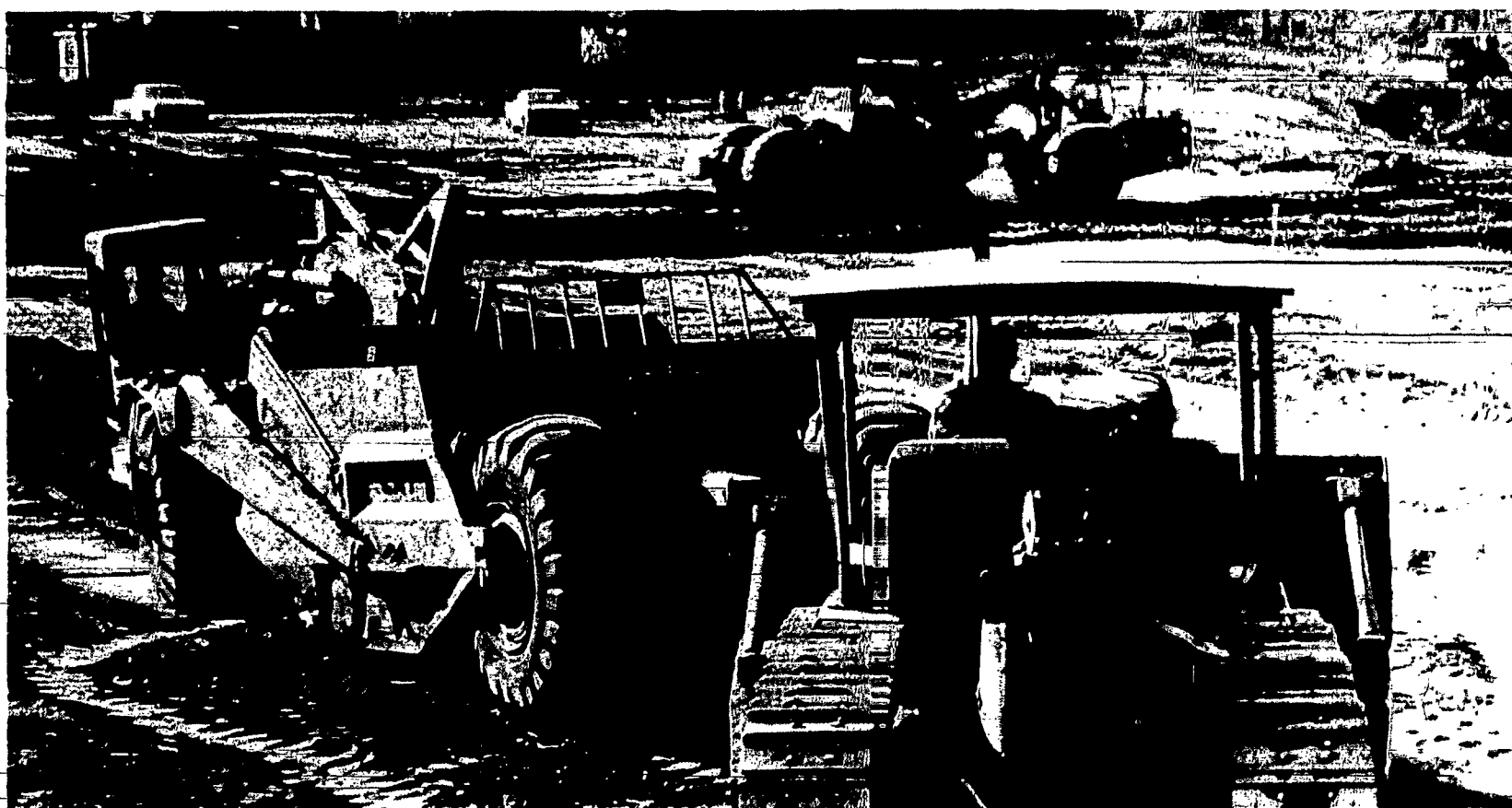
Earth-movers etched the outlines of new Becket Hall, residence for seminarians at St. John Fisher College Druid Hills campus south of Fairport Road in the town of Pittsford.
