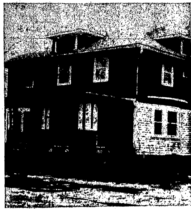
This will be the new rectory of St. Patrick's parish at 46 Stanley St., Mt. Morris. The former D. F. Russell home, recently purchased, is being enlarged and remodeled.
