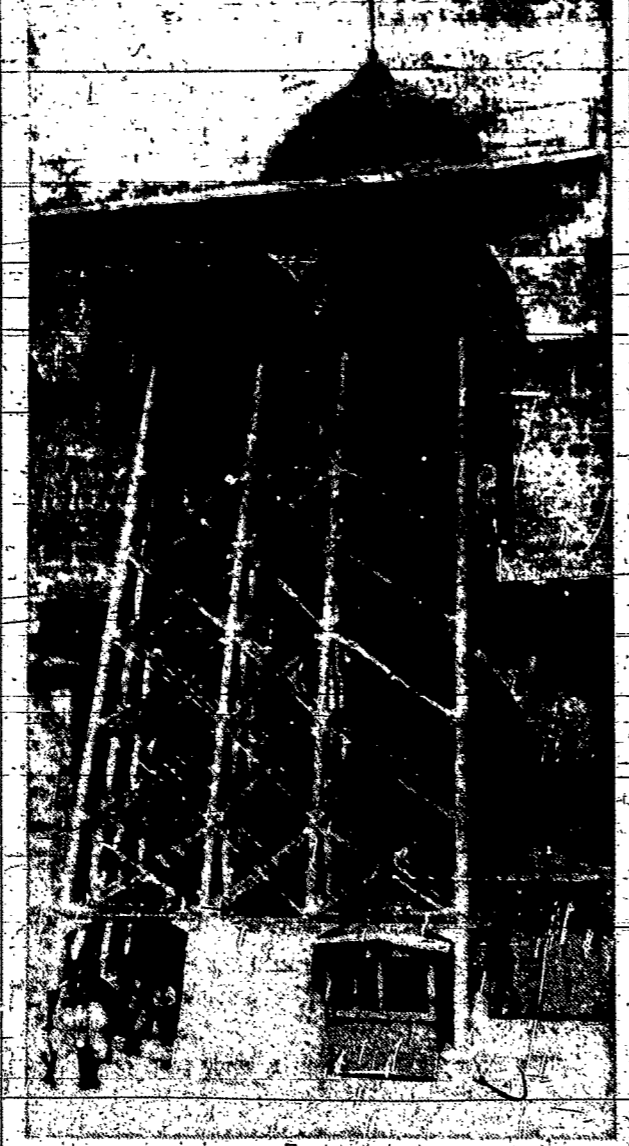
The Holy Sepulchre basilica, a hodge-podge of centuries-old structures, is shored up by steel and massive wood girders, a sorry spectacle for pilgrims who come to the site where Christ died and rose to eternal life.
