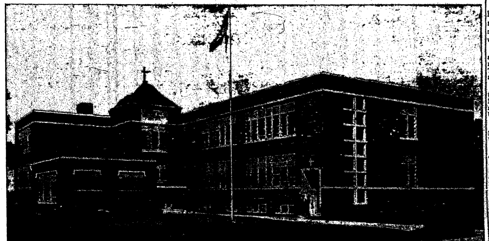
Artist sketch of proposed new St. John the Evangelist School, Humboldt St., Rochester.
