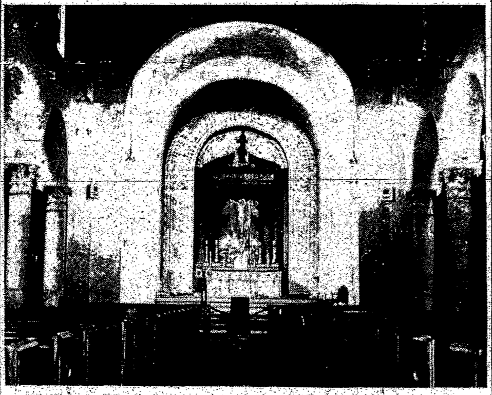
St. Francis Church, Phelps, where golden jubilarian Father Simpson has been pastor for 40 years. He supervised church design and construction in 1931.
