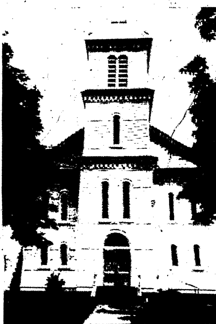
APPROACHING Perkinsville Church
