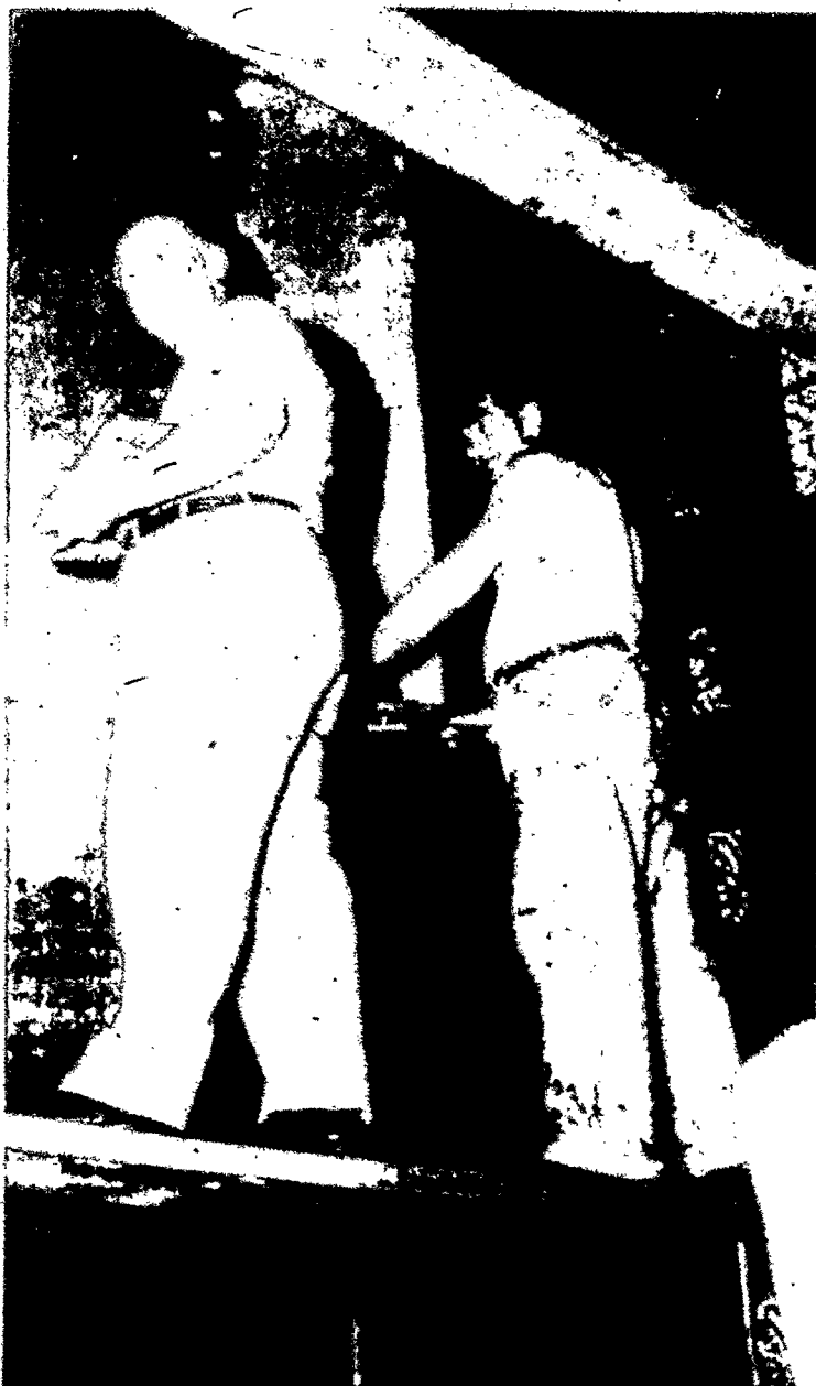
ST. BERNARD'S seminary chapel is currently undergoing a complete renovation. Workmen are shown decorating new niche above main altar for statue of the Blessed Virgin Mary.
