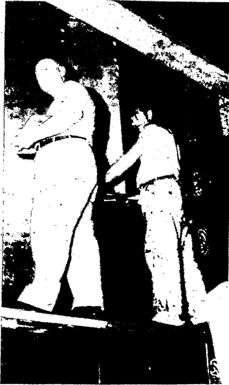
ST. BERNARD'S seminary chapel is currently undergoing a complete renovation. Workmen are shown decorating new niche above main altar for statue of the Blessed Virgin Mary.
