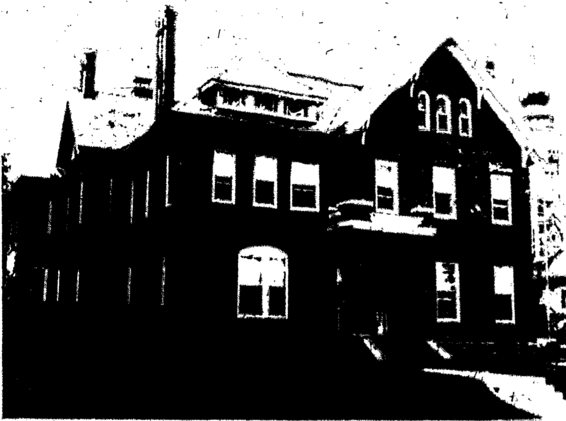
CONVENT at Holy Redeemer Parish was given a face lifting, both inside and out in general repair work done recently on the parish property.
