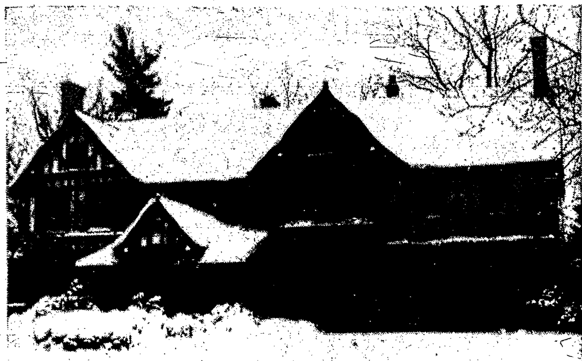
NEW GIRLS' HOME — The Walter Todd residence (above) at 1475 East Avenue will become the new St. Elizabeth Guild House, a diocesan-operated home for young working women. The present Guild House, located at 1 Field Street, will be razed to make way for construction of the new Eastern Thruway feeder.
