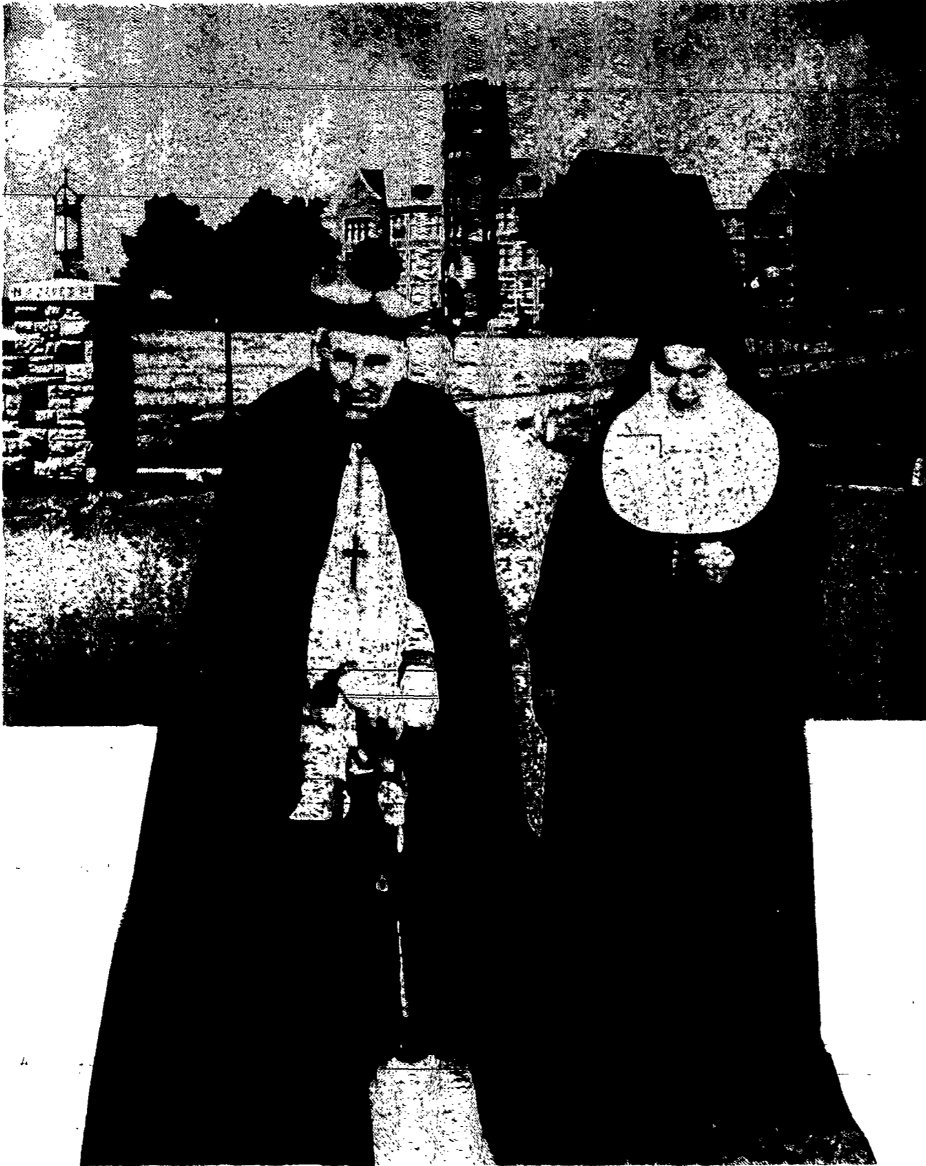
Breaking ground for new construction of Nazareth College.
