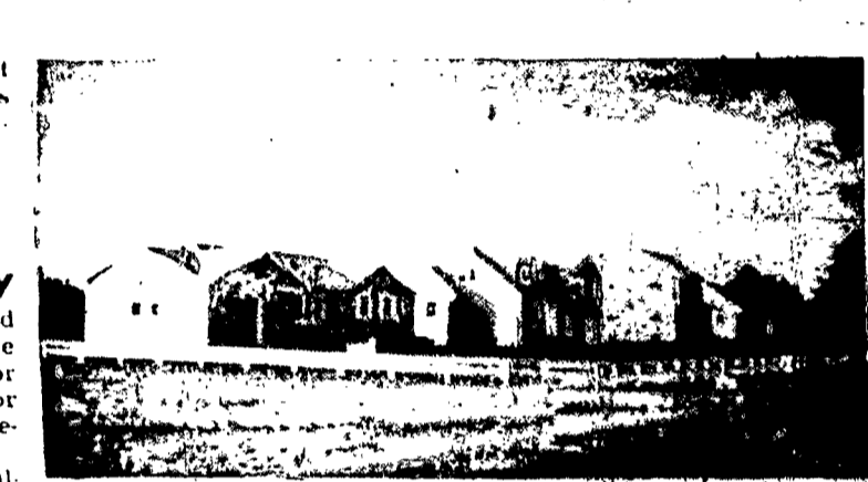
"South Ridge Estates" new construction. Pepperidge Homes, bldrs., St. John's Parish.
