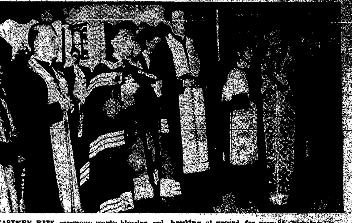
EASTERN RITE ceremony marks blessing and breaking of ground for new St. Nicholas Ukrainian Catholic Church in Elmira Heights. With Bishop Ambrose Senyshyn. (second from left) taking part are: (from left) Very Rev. Basil Seredovich, Syracuse; the Very Rev. Nicholas Wolensky, Rochester, and the Very Rev. W. B. Dowhovitch, pastor of St. Nicholas.
