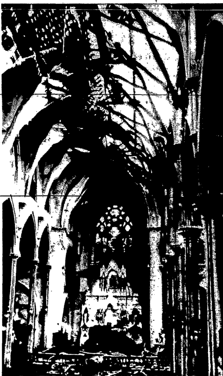
PRE-DAWN FIRE — Interior view shows results of a pre-dawn Sunday fire at St. Patrick's Church, Hartford, Conn. For a time the 14th floor was in danger of toppling but building inspector states church is repairable. Damage was estimated at $200,000. The blaze was the first of two church fires in Hartford, the second destroying St. Joseph's Cathedral. (NC Photos)
