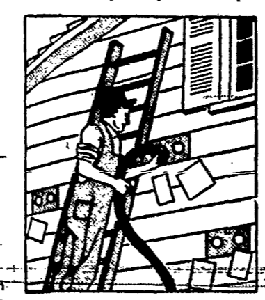
Installing mineral wool.
